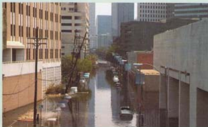
Levees and floodwalls were meant to protect New Orleans from rising water levels. However, after Hurricane Katrina, these barriers broke, flooding the city and submerging homes, buildings, and cars.
