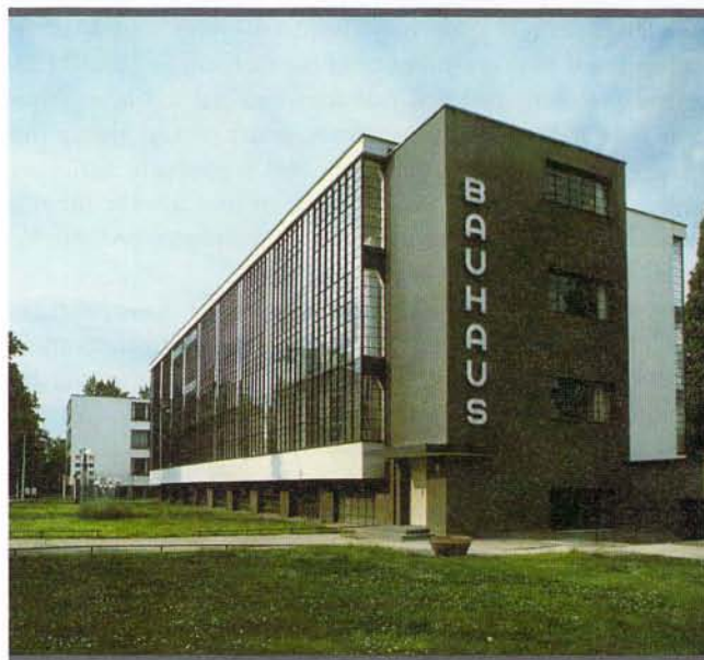
Walter Gropius, The Bauhaus. Walter Gropius was one of Europe’s pioneers in modern architecture. When the Bauhaus moved to Dessau in 1925, Gropius designed a building for its activities. His straightforward use of steel, reinforced concrete, and rows of windows reflects the move to functionalism in modern architecture.
