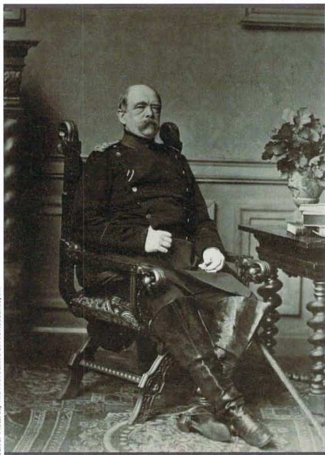
Culver Pictures/The Art Archive at Art Resource, NY
